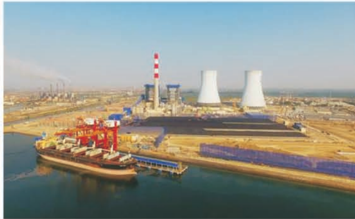
Project : Pakistan Haveli Power Plant Model & Units : R-C2200S/R-DC500S * 3 City : Pakistan
